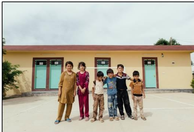
Hasira Secondary School Expansion
